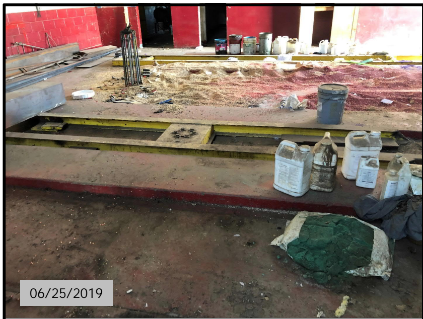
PHOTO 9: Belowgrade hydraulic lifts located within the eastern building at 225 North Harris Street
